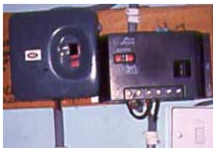
Figure 7: A by-passed charge regulator. (Photo from field study)
